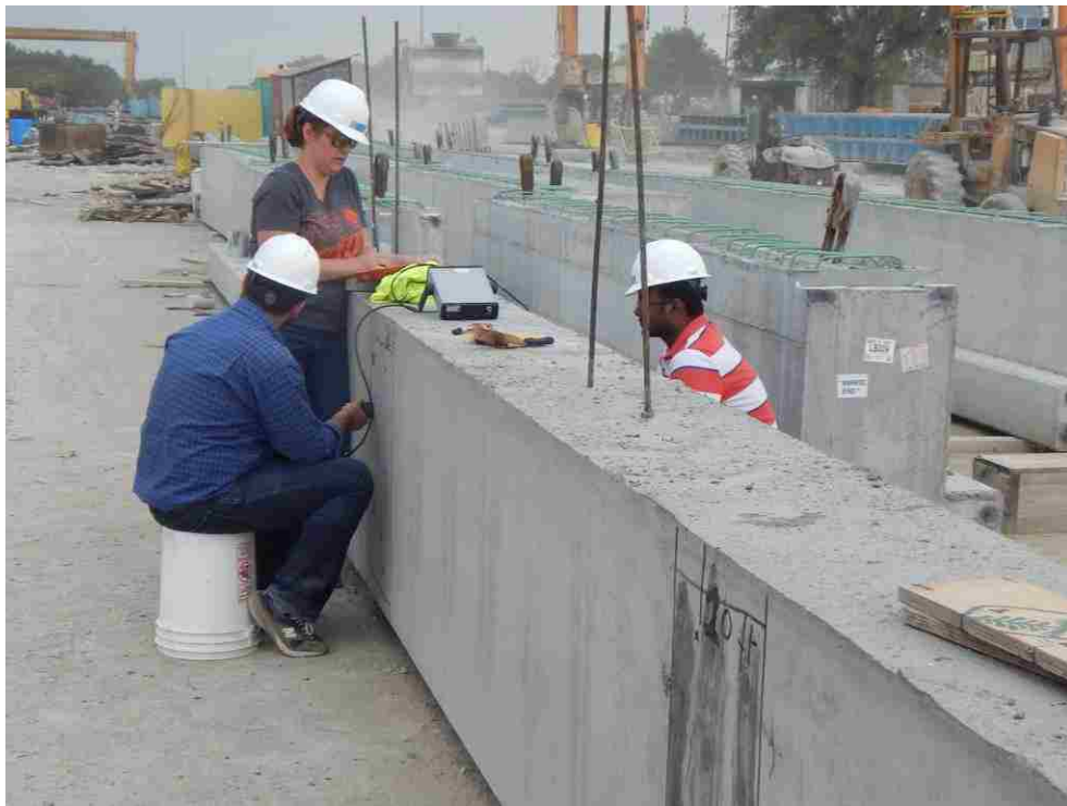
Figure 5.21 On-site UPV testing on beam.
