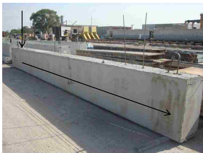
Figure 5.7 Beam 5 with the three sets of pre-stressed strands. The arrows indicate the direction of casting.
