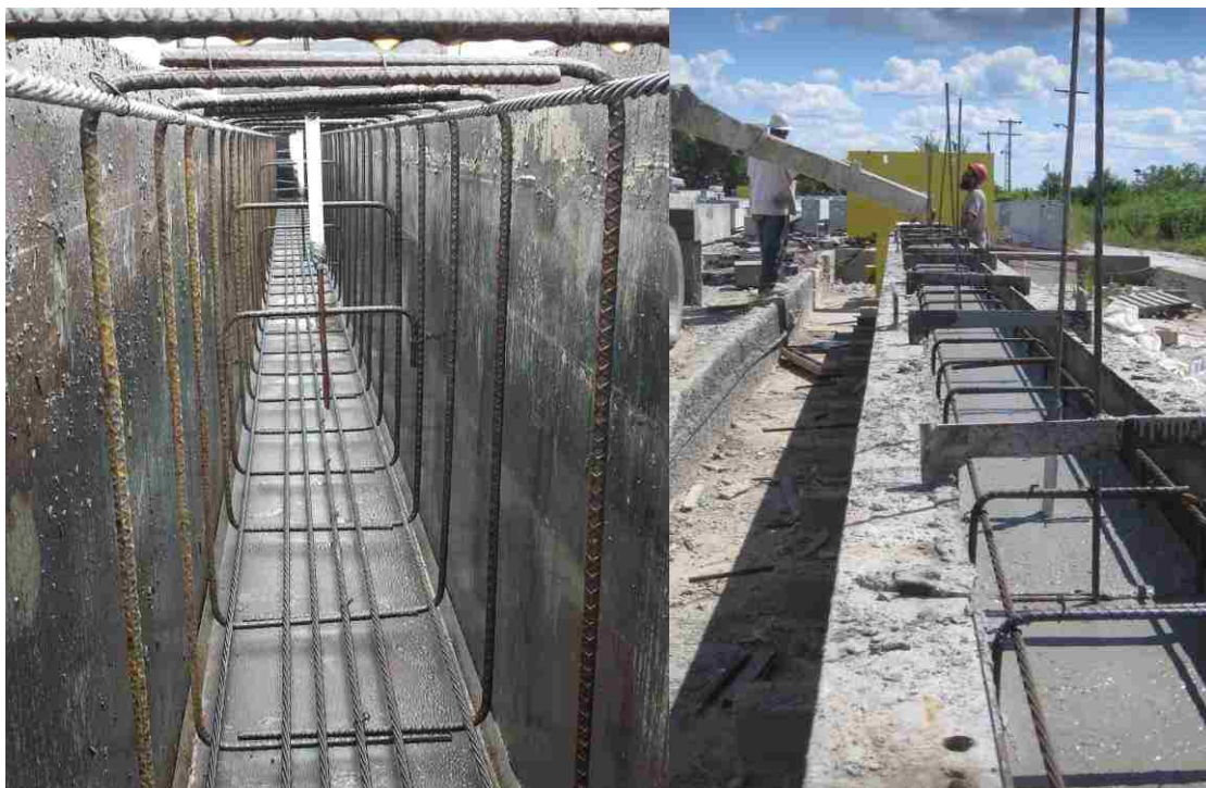
Figure 5.5 Left: Reinforcement of the rectangular beams. Right: Casting beam.
