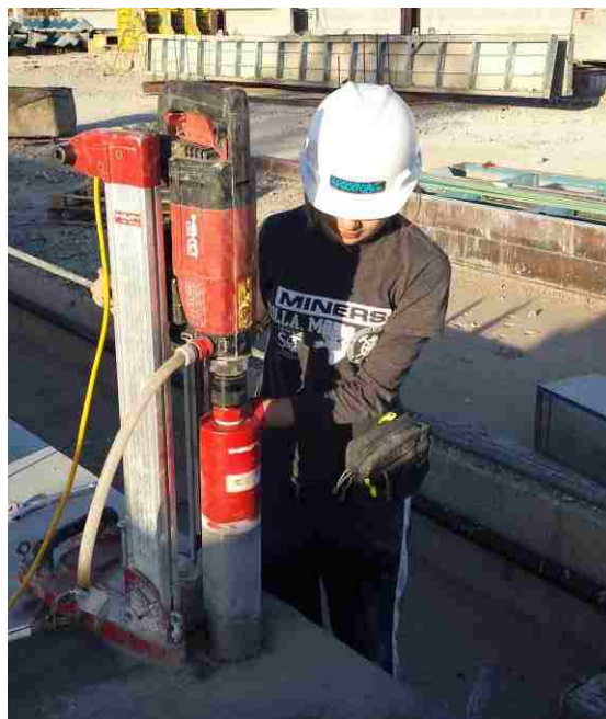
Figure 5.18 Extracting cores from a beam.
